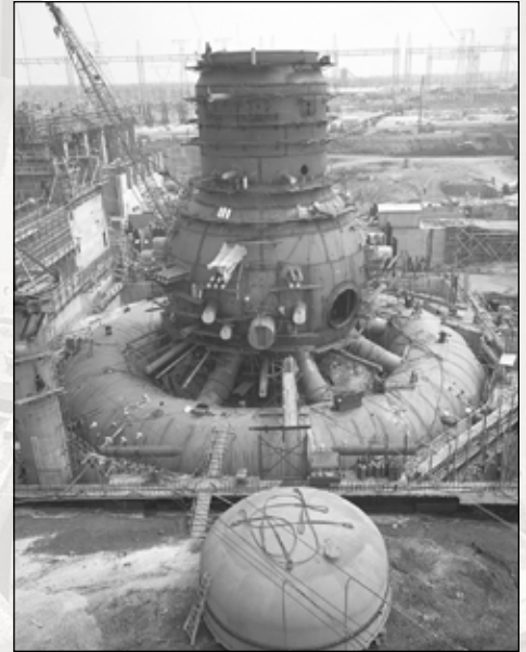
Brown's Ferry Unit One under construction.
